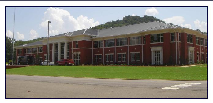
The 87,462 square foot impressively designed building called for a variety of construction methods including concrete monumental stairs, both wood and metal framing, pre-engineered metal building, metal roof, and a building-wide hollow core concrete slab for the 2<sup>nd</sup> floor.
