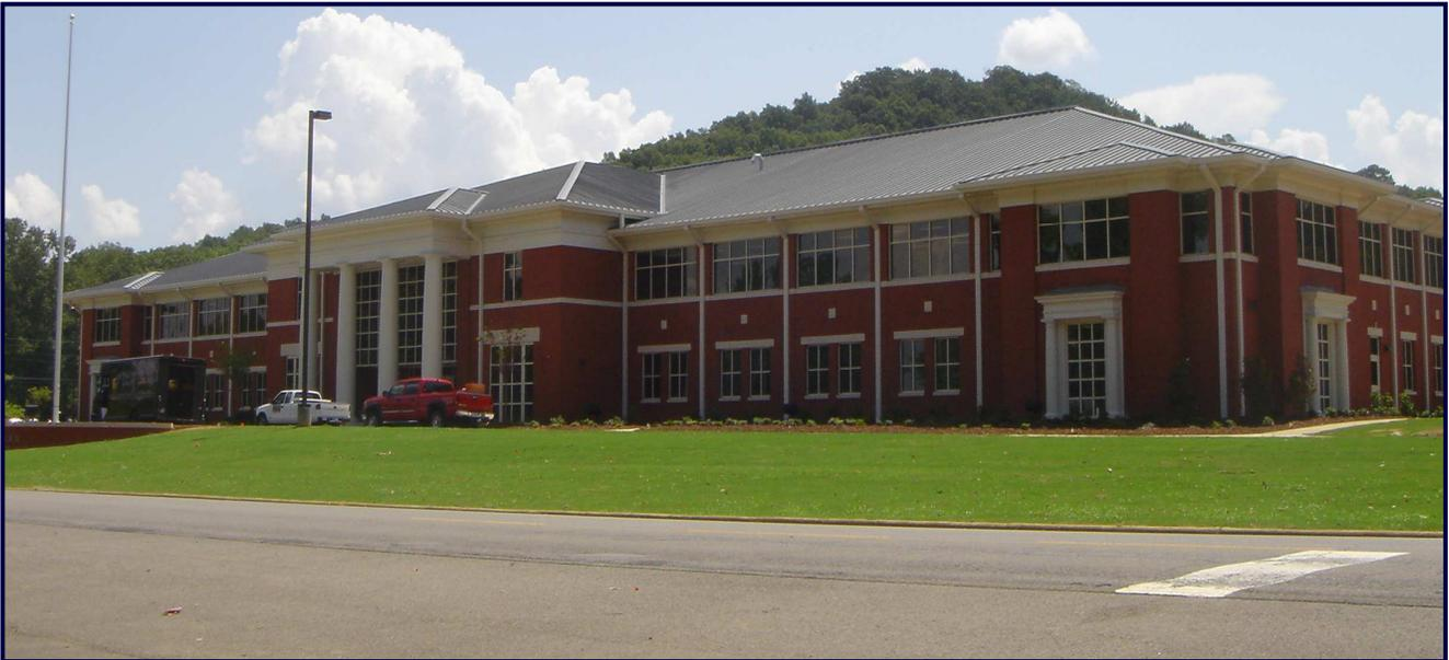
The 87,462 square foot impressively designed building called for a variety of construction methods including concrete monumental stairs, both wood and metal framing, pre-engineered metal building, metal roof, and a building-wide hollow core concrete slab for the 2<sup>nd</sup> floor.
